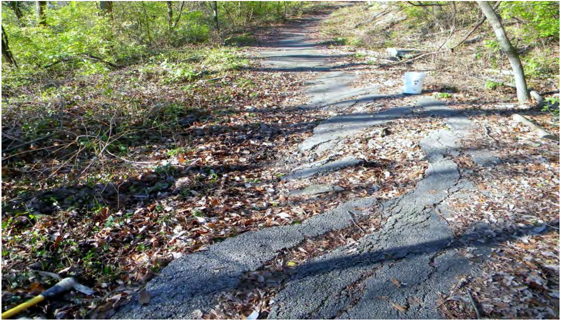
Figure AV.8: Scarp face of one of the landslides at the Delhi Pike landslide complex site.
