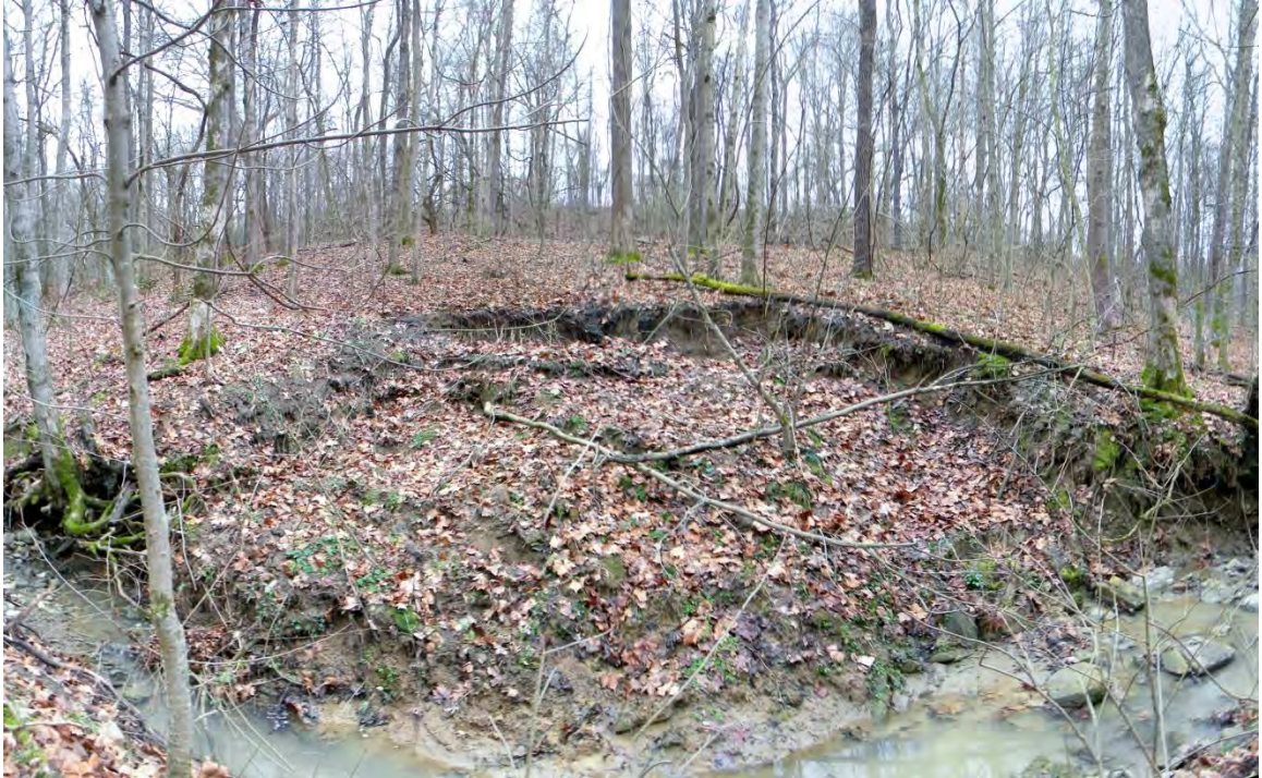
Figure AV.18: Scarp and toe the Old US52 landslide. Notice the small stream undercutting the toe.
