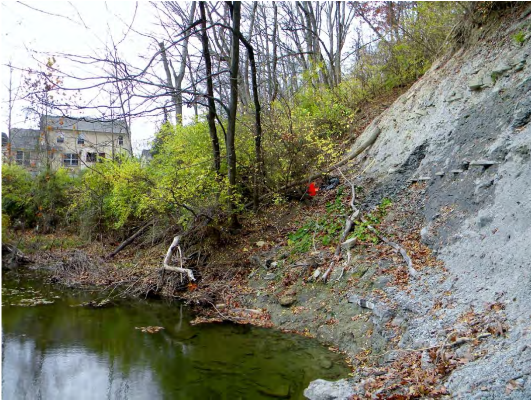
Figure 6.11: Undercutting the toe of the slope at the Berkshire Road landslide.
