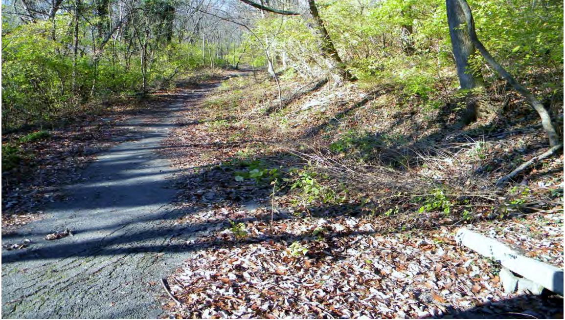
Figure AV.9: Toe of one of the landslides at the Delhi Pike landslide complex site.
