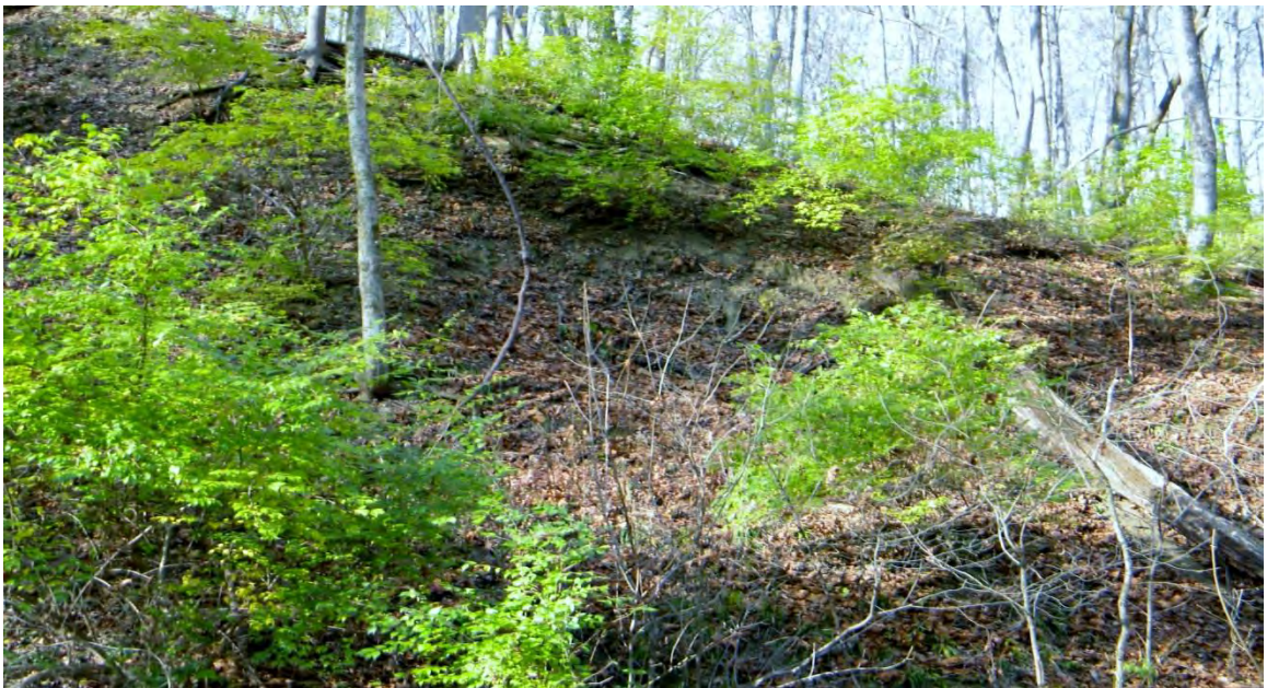
Figure AV.15: Head scarp of the Nordyke Road landslide.
