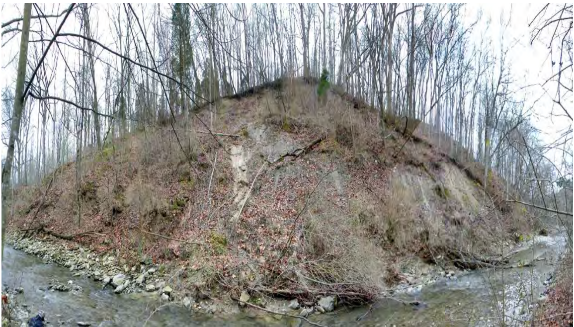
Figure AV.5: The toe of the Ten Mile Road landslide, undercut by a stream.
