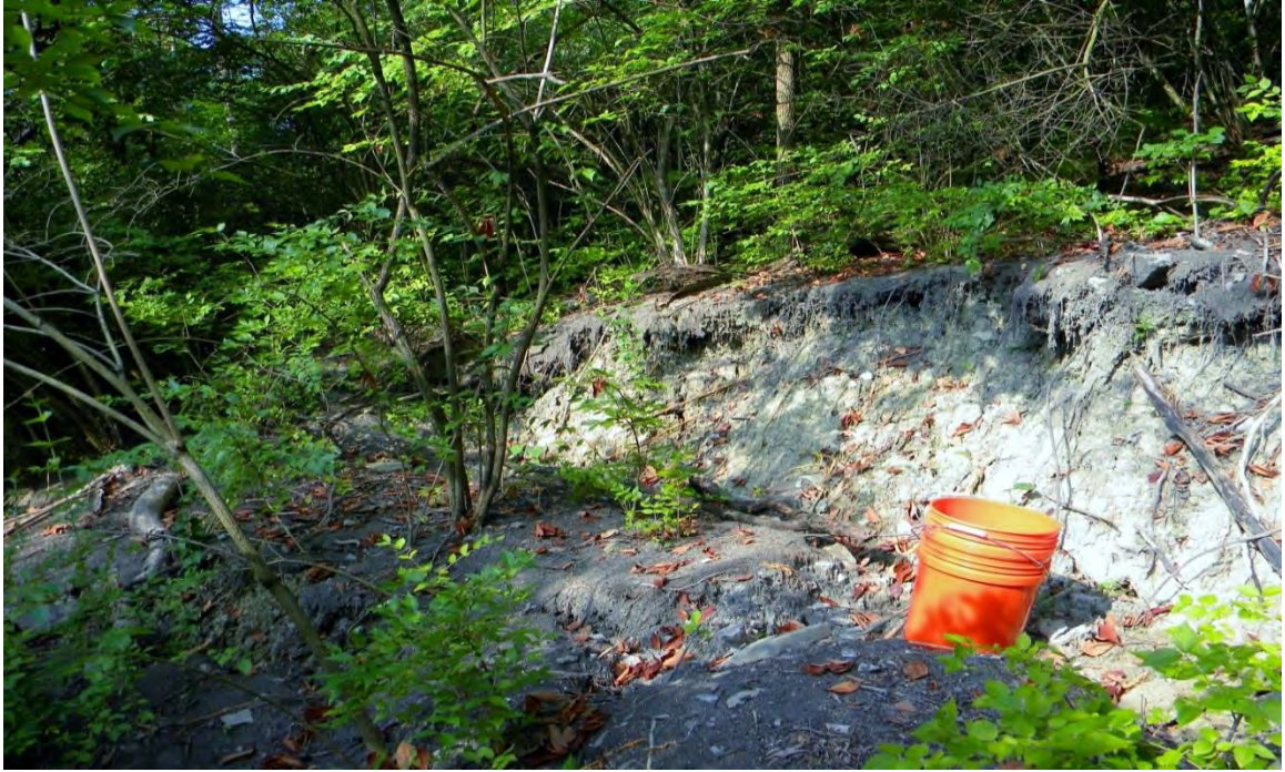
Figure AV.28: Head scarp of the Columbia Parkway landslide.
